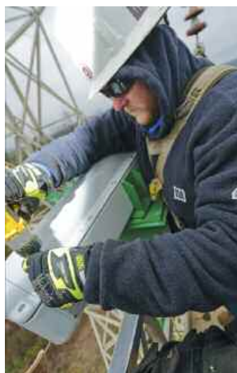
Swafford secures one of 20 bolts that hold a new transmission device, the DSR.
