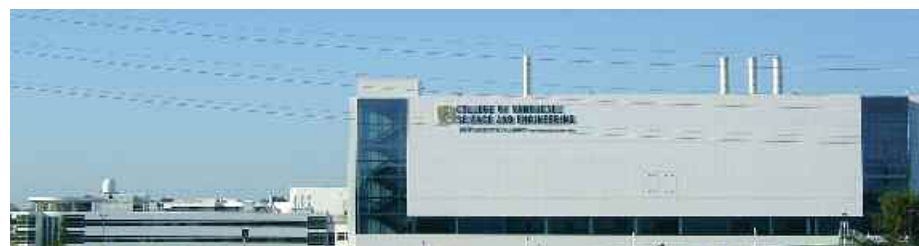
A Local 236 project, NanoFab X at the College of Nanoscale Science & Engineering, University at Albany, was recently completed.
