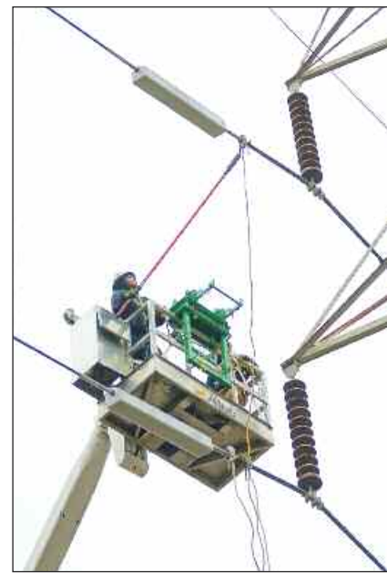
The DSR installed on 161-kilovolt transmission lines owned by the Tennessee Valley Authority
